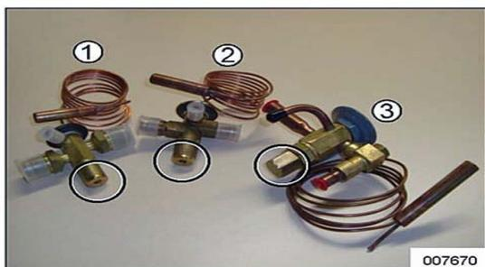
The adjusting screw of expansion valves types (1) & (2) is located under a Allen head plug, expansion valve (3) is under a hexagonal cap.
